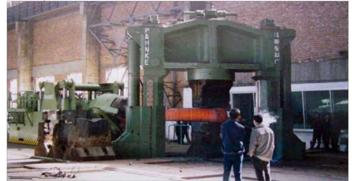
30 MN forging press, Simmaco, Bao Tou (same construction as QSP)
