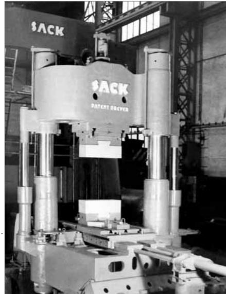
10 MN open die forging press, Schoeller Bleckmann, Ternitz, Austria
